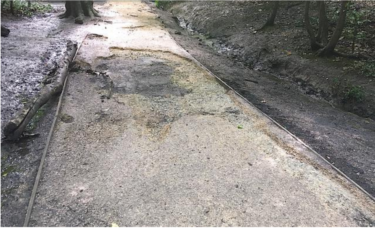
9 Next morning. The aggregate surface of the path above the Frogpool had been washed away into the stream and its gullies.
