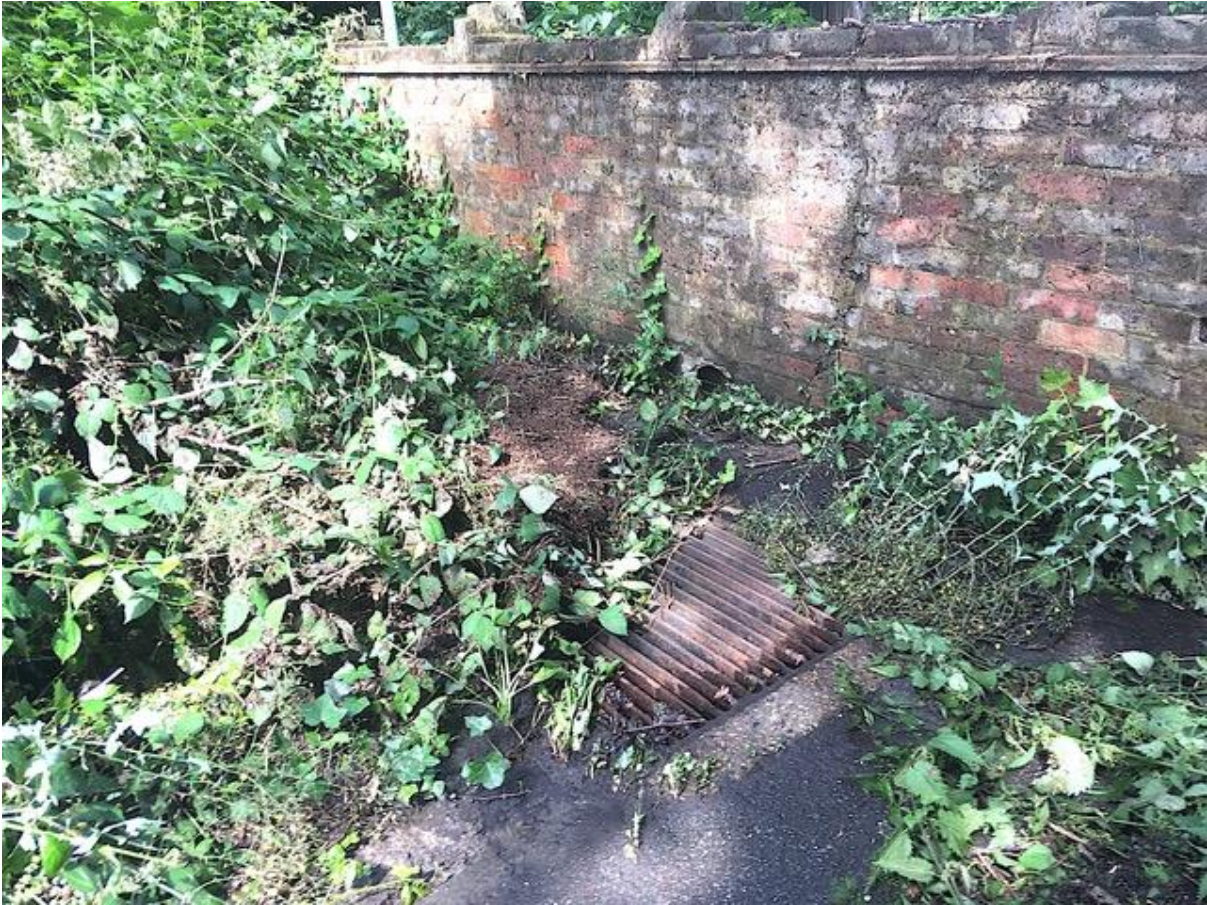
5. Next morning. This shows the Wood Vale entrance wall and inlet grating. The wall is undamaged. Vegetation has been flattened, and has silt on it. There was silt and debris in and around the grating.
